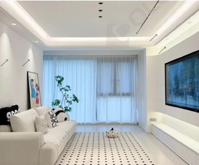
There is color inconsistency between vertical light troughs and ceiling light troughs.
