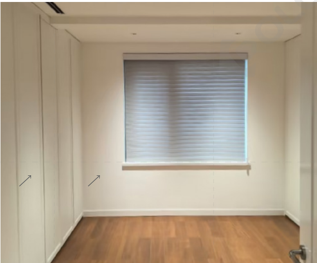
There is a color difference in the lighting between the two vertical walls.
